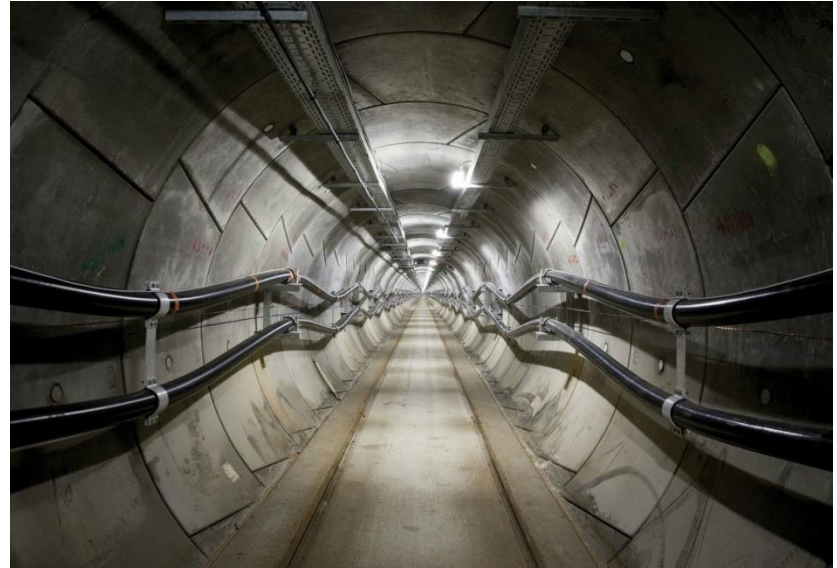
Tunneling under the Alps for the France – Italy interconnector
